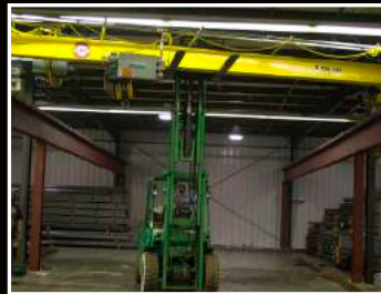
Bridge Crane Installation
